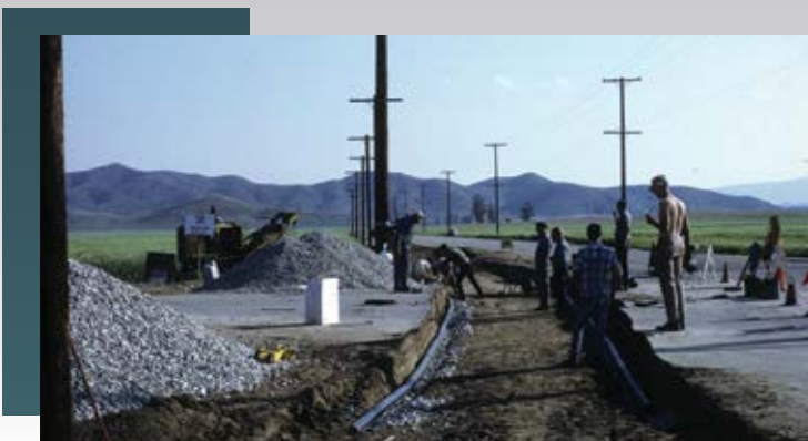
Figure 19-06: On April 6, 1968, a museum team prepares the recently dug trench across Mapes Road to receive a load of rock ballast. Drain pipes have already been installed along both sides. The view is south. (SCRM Archives/Jim Walker photo)
