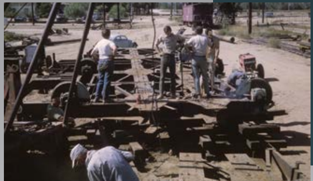
Figure 19-05: A team of museum members works to reassemble the transfer table that was salvaged from the PE Torrance Shops. The scene is between the current Carhouse 1 and Carhouse 3. (SCRM Archives/Jim Walker photo)
